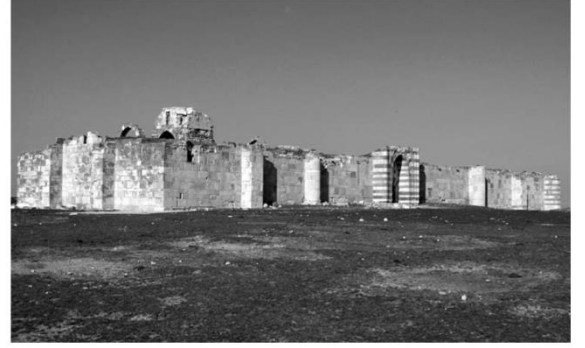
Fig. 4 Sadeddin Han, South and west facades. Source: M. Önge photo archive.
